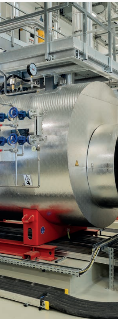
A total of five electric boilers for steam generation (left) have been installed at the Kundl (top) and Schafftenau (bottom) sites over the past few months.
